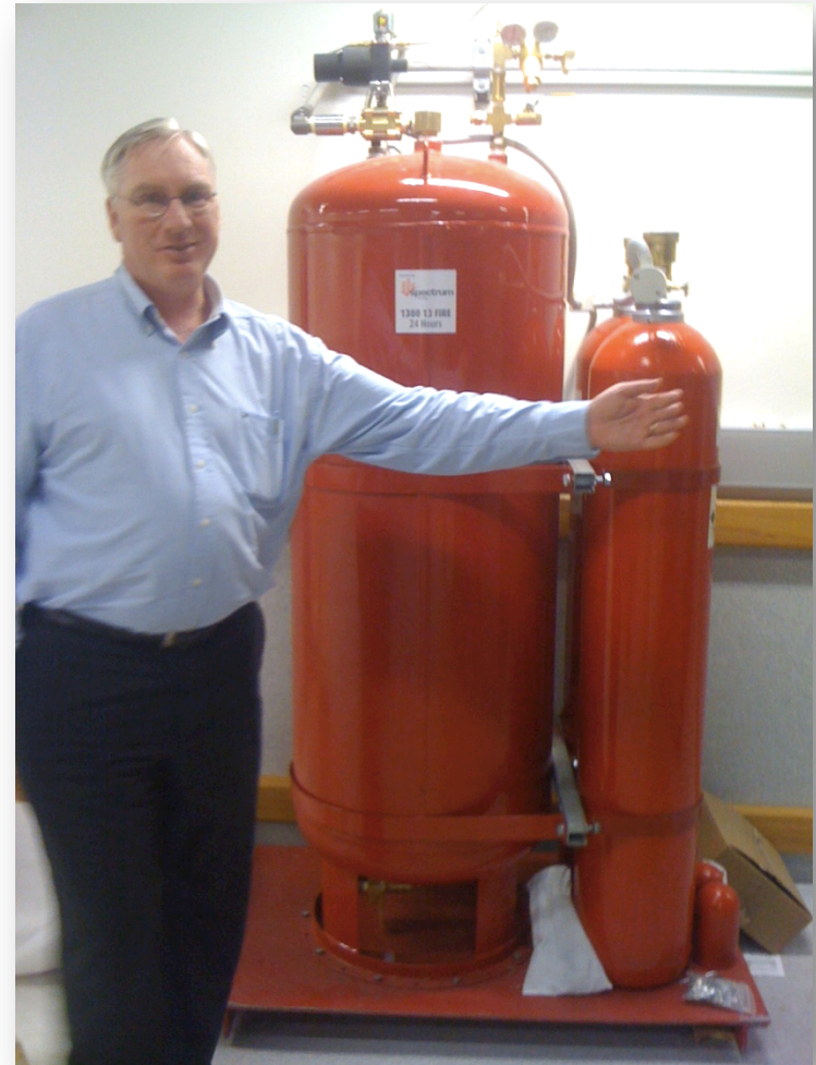
Mark Fisher-Chief IT Architect with nitrogen discharge water mist fire suppression system
