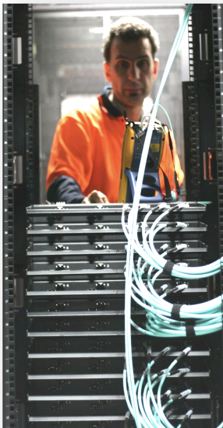
Installation Engineer, cabling the Ampnet fibre distribution in the new R1 data centre
