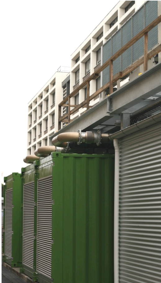
Three 450KvA generators at the rear of the new R1 Data Centre
