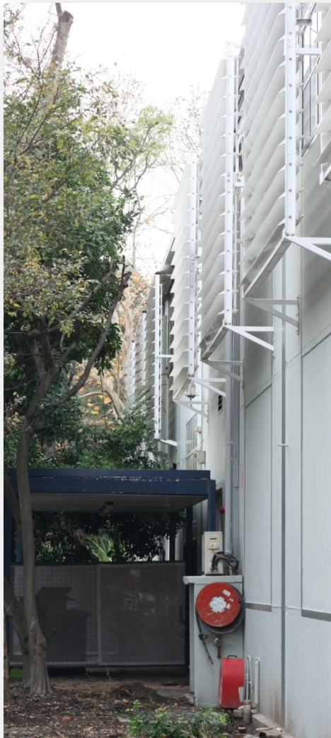
Front entrance to the new R1 Data Centre
